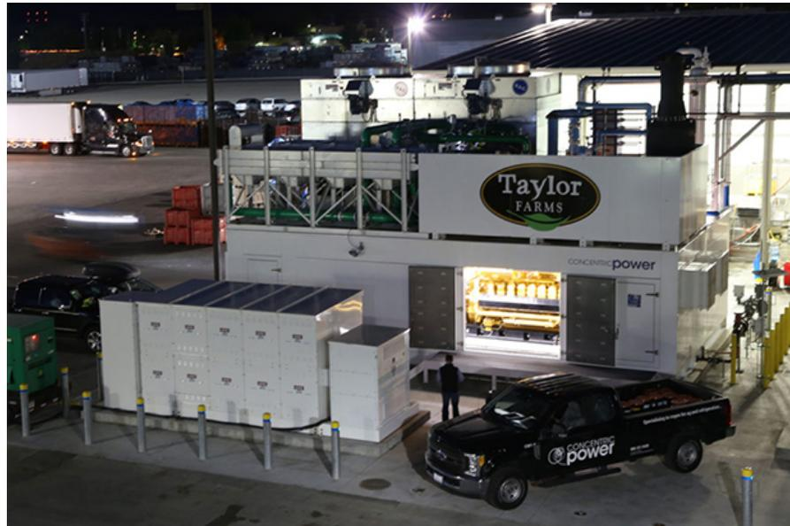
1. Concentric Power supplied a 2-MW natural gas-fueled power system with cogeneration capability for a Taylor Farms facility in Gonzales, California. *Courtesy: Concentric Power*
